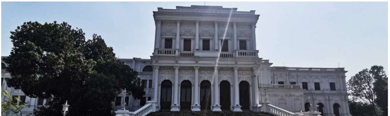
Belvedere House, National Library, Kolkata; Source - DRONAH
