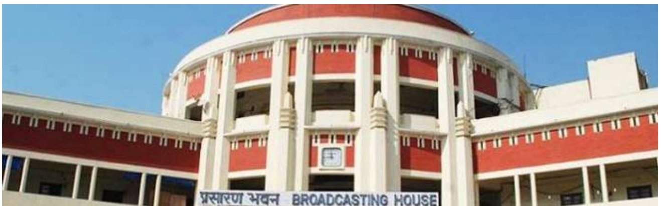
All India Radio - Prasar Bharti Building; Source - preasarbharati.gov.in
