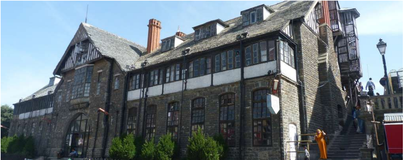
Town Hall, Shimla; Source - DRONAH
