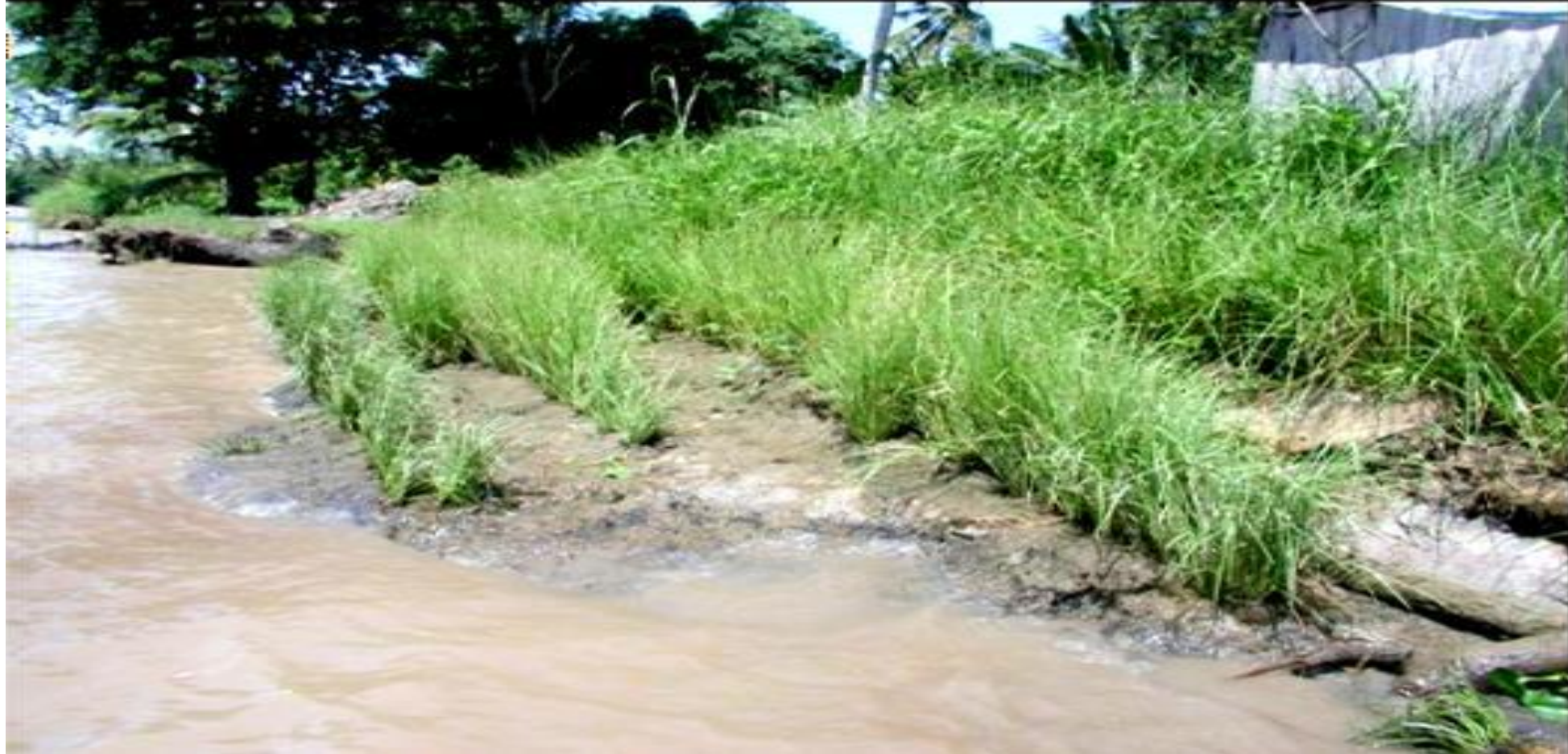
Mekong Delta Vietnam: Protecting bank against wave erosion
