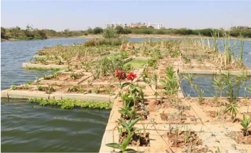
**Figure 4.2.4:** Floating treatment wetland at Nekkampur Lake, Hyderabad
