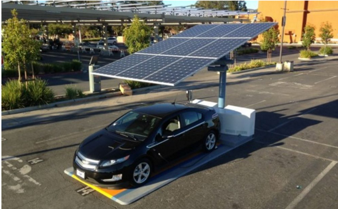
Figure 9.7: Off grid solar EV charging station in California
