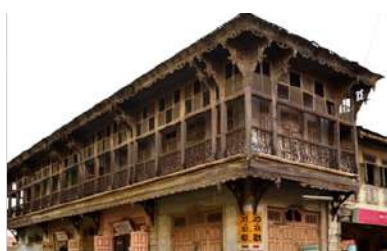
Islamic Heritage building, Rander, Surat
